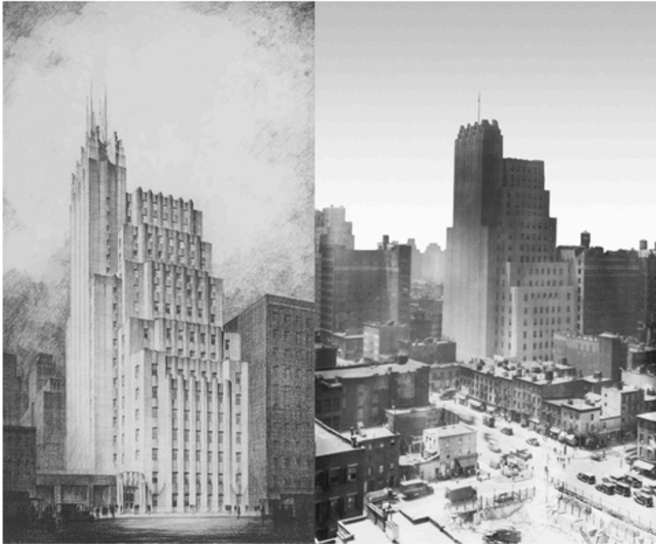
At left, a preliminary drawing of the Telephone Building at 212 West 18th Street from the late '20s. The building at completion, photographed in 1931 (at right), which shows the lack of a full-height spire, something the Walker Tower developers are planning to add back at penthouse level.
